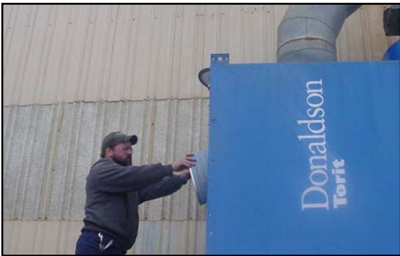
Donaldson Torit Ultra-Web filters have given Ready Machine Tool & Die Corp 4-times longer filter life and significantly improved air quality inside the plant.
